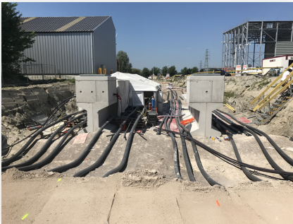
Installation cable system
